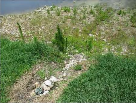
ii. Step erosion was observed on the northwest bank of lake 36 that should be monitored.
