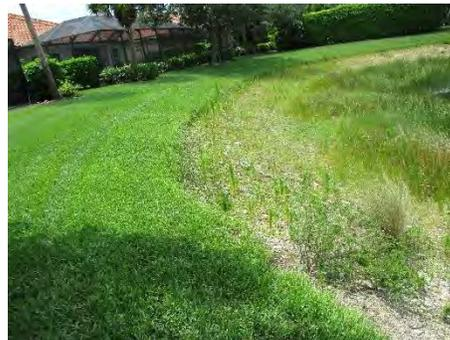
iii. The Board may wish to consider having a drain added to the cart path at the low point adjacent to 9184 Quartz Ln. as erosion is beginning to develop and it appears it is developing from the cart path runoff.
